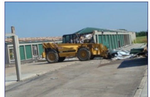
Jim Gollither performing demo work for CRI on SR 31 in Kokomo
