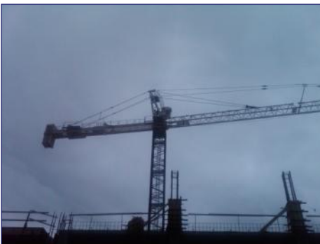
Mike Thurman working for Wilhelm at IUPUI parking garage.
