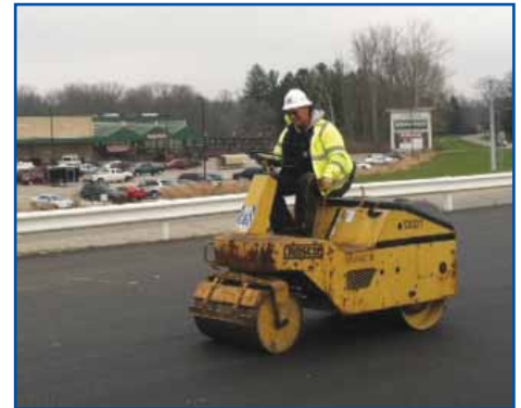
Jerry Wilson rolling a parking lot in Richmond
