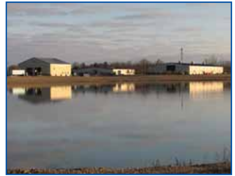
Apprenticeship & Training Facility with new shop
