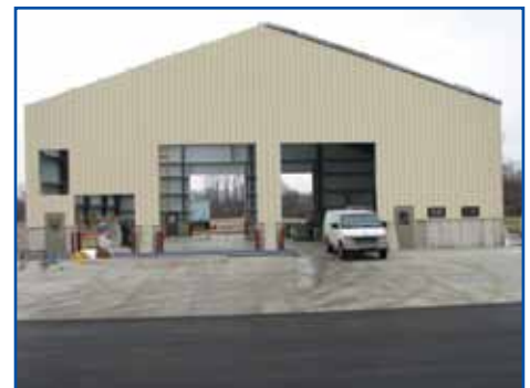
View of new shop from the main office 10-30-11
