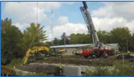
Calumet working on S.R. 28 in Albany
