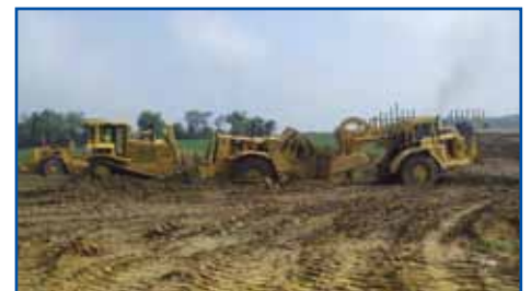
Fox working on US 31
